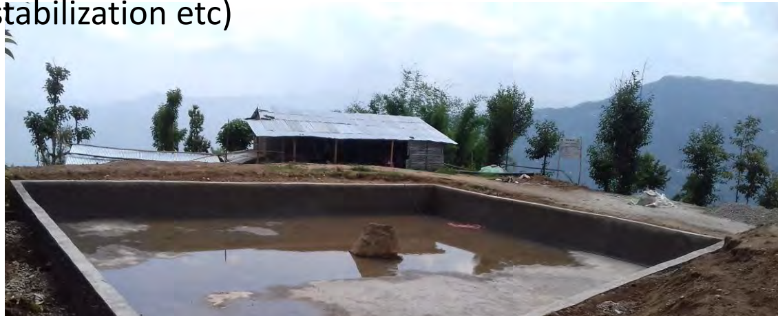
Pond in Betali VDC, Ramechhap to collect excess storm water to reduce soil erosion and to use for agricultural purpose under USAID_Sajhedari_Bikaash_Project
