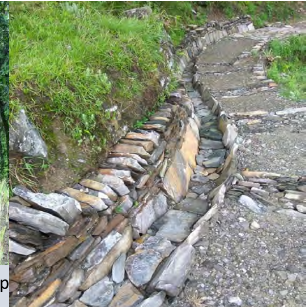
Low cost drains constructed under Unnat Goreto along the trails
