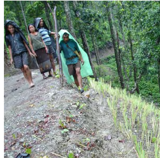
Bio engineering added in a road p Food for work project
